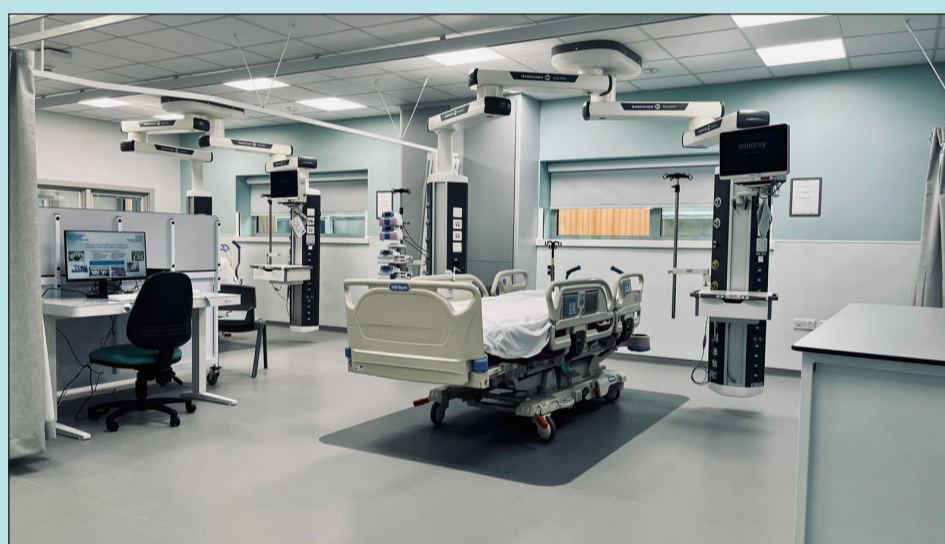
Bed-bays at the new Intensive Care Unit (ICU)
